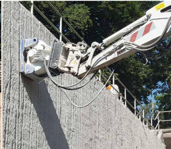
▲ A **DMW220** cuts through 60 cm thick concrete slabs at a rate of 1.5 m/min. The concrete contained re-forcement with diameters from 16 mm to 25 mm. The wheel cut through all of the steel bars without any problems.
