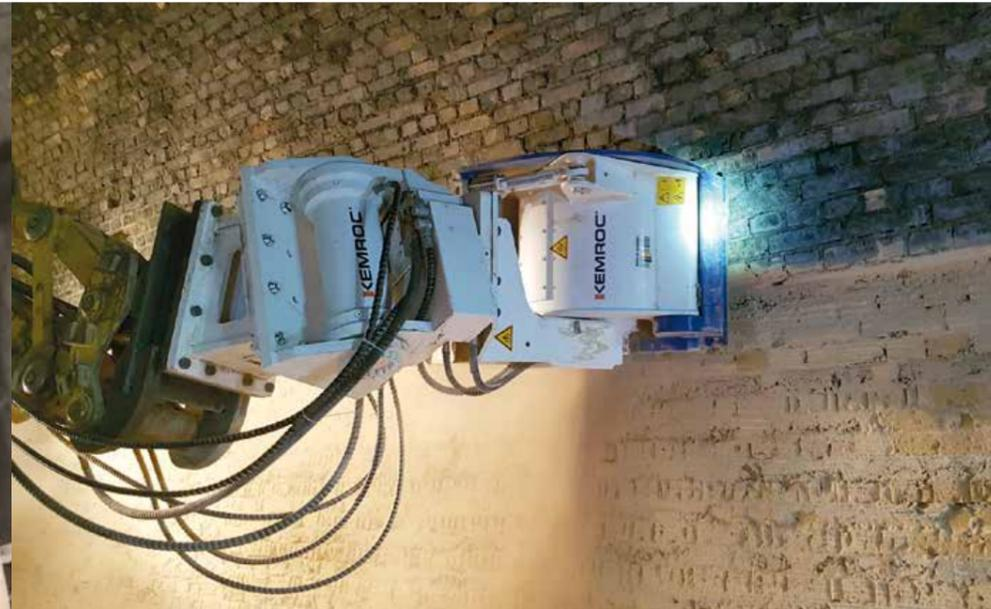
▼ An **EK140** chain cutter lowering a tunnel floor in fine grained gneiss.
