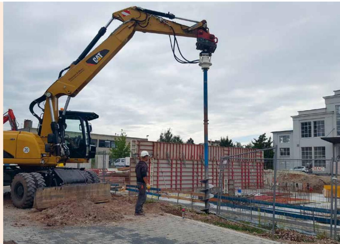
▲ An **EBA2300-D** drilling 5 m deep holes for the installation of steel piles that will be required for the construction of a retaining wall.
