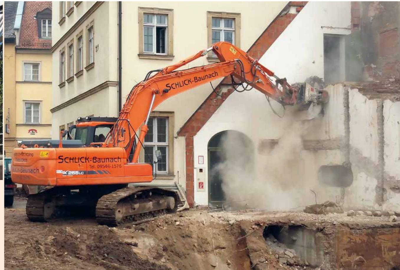
▲ A low vibration **DMW130** cutter wheel used to demolish part of a wall. Part of the wall could be demolished without damaging the rest of the wall or the historical building that it was attached to.
