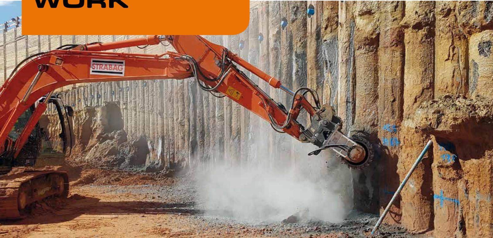
▲ The surface layer of concrete drill piled wall are profiled to a high degree of accuracy using an **ES60HD** fitted with a cutter drum.
