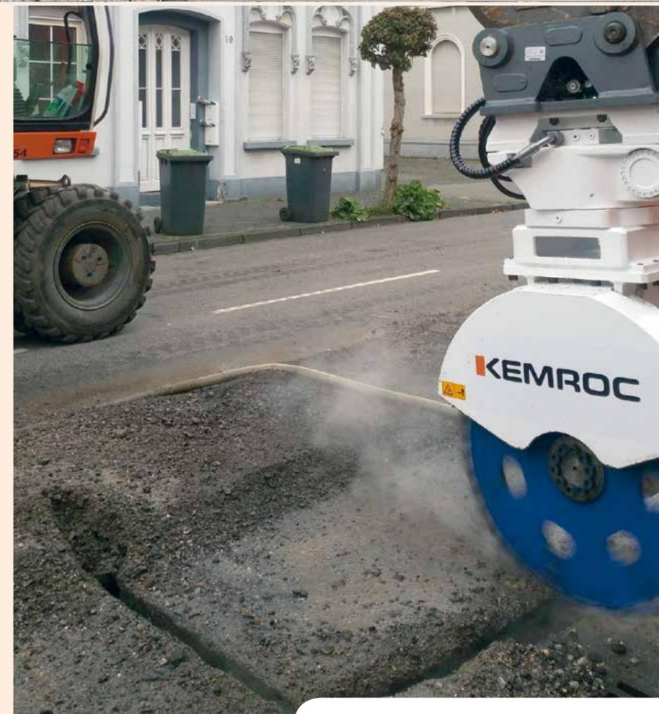
▶ An **ES60HD** with rotation unit mounted on a Liebherr A 900 wheeled excavator cuts through a 30 cm thick asphalt layer. The cutting speed is 2 m/min.
