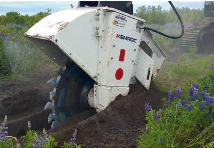
▲ In Iceland, this **DMW 220** cut a 70 cm deep by 15 cm wide slot for cables in lava rock. The production rate was around 30 meters per hour.
