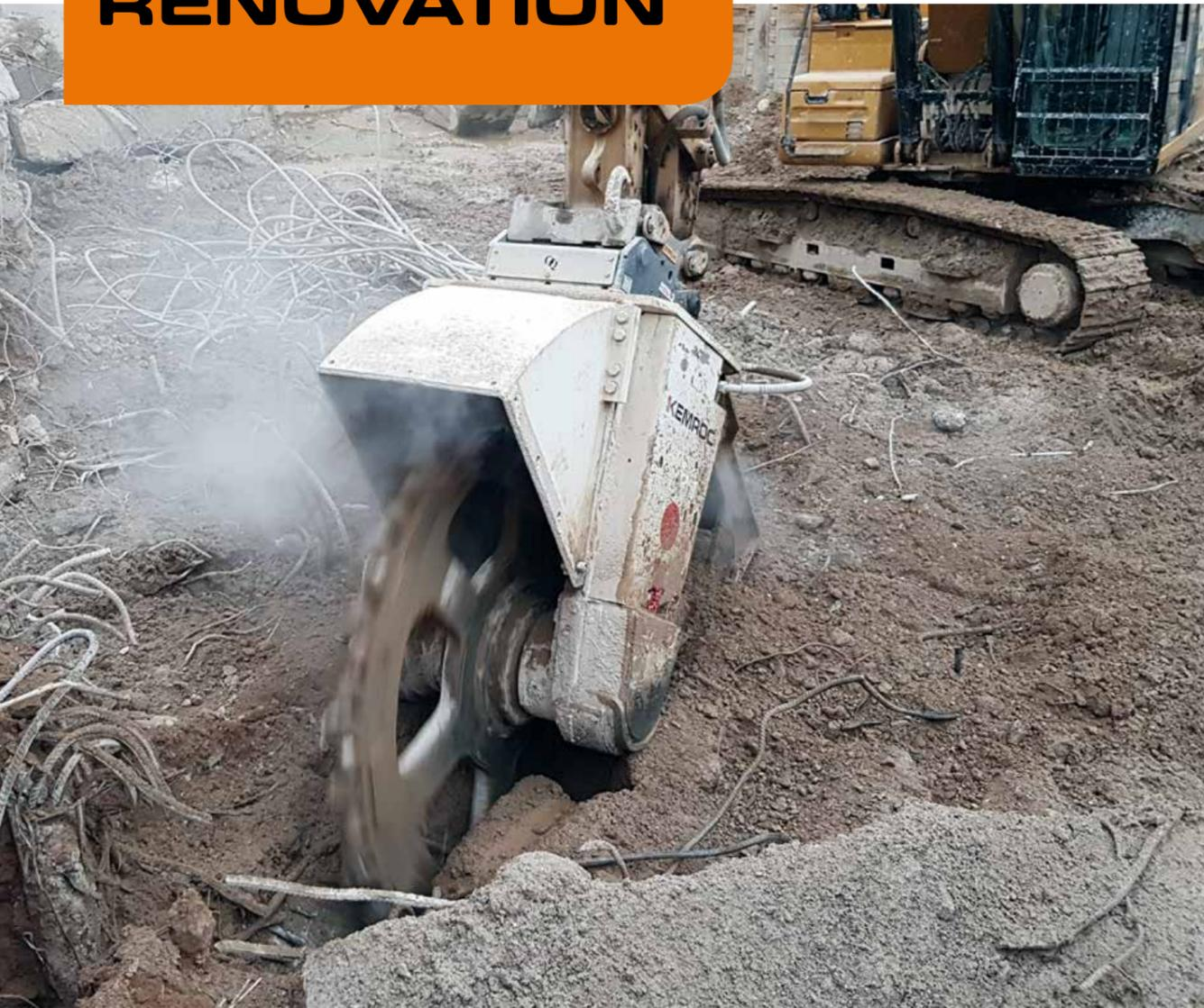
▲ A **DMW220** cutter wheel being used to cut through a 900 mm thick concrete floor containing 30 mm diameter rebar laid in a tight pattern.
