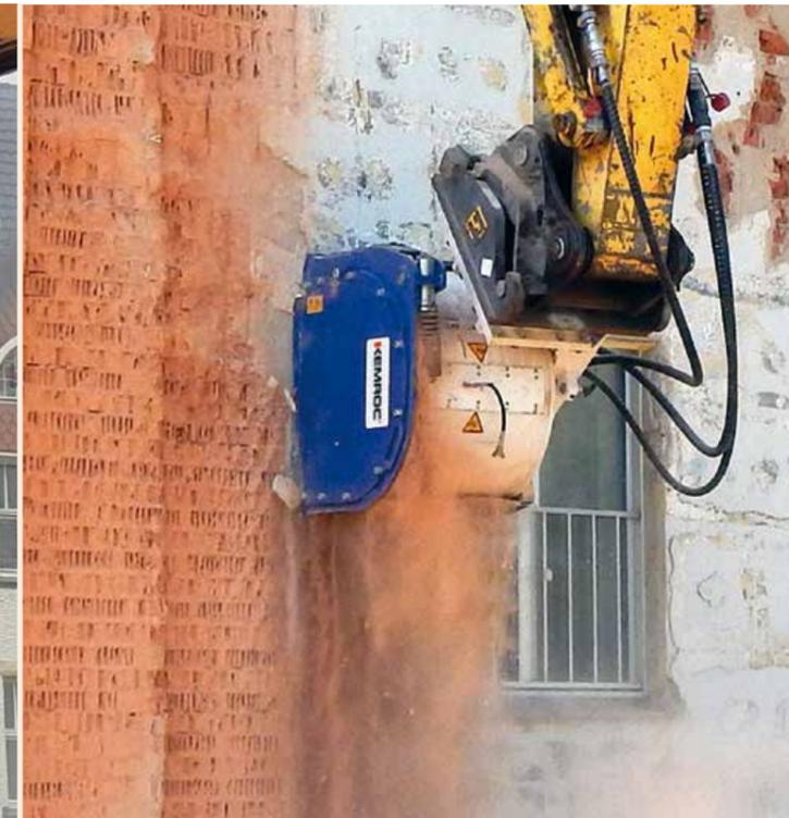
▲ At an old barracks building, a contaminated layer, 50 mm deep, had to be removed before the remaining building could be demolished. The maximum operating height was 25 m and the production rate for the **EX60HD** was 5 min for 12.5 m<sup>2</sup>.
