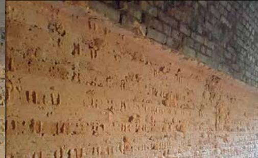
▼ Cutting 60 cm deep de-stressing slots with a **DMW130** cutter wheel so that the concrete segments can be broken out with a ripper tooth at a later stage.
