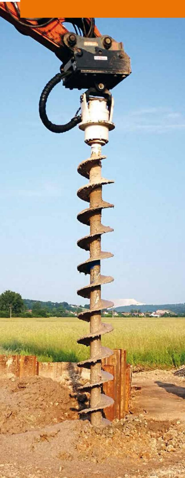
◀ An **EBA2300-D** drilling holes to 6m depth in medium hard ground to loosen it up and make the ramming of piles easier.
