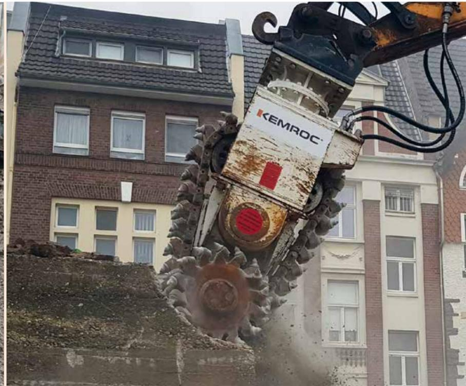
▲ Demolition of a bunker using an **EK140** chain cutter. The bunker is attached to another building and a low vibration method must be used to demolish it.
