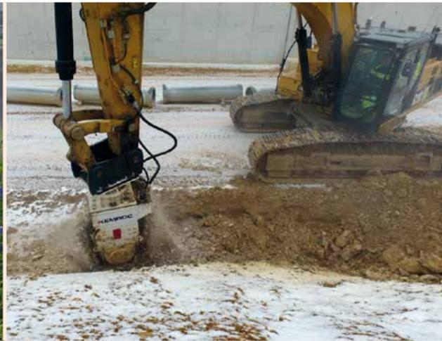
▲ This **EK 140** was used to excavate drainage channels at the foot of an embankment close to an ICE train line.
