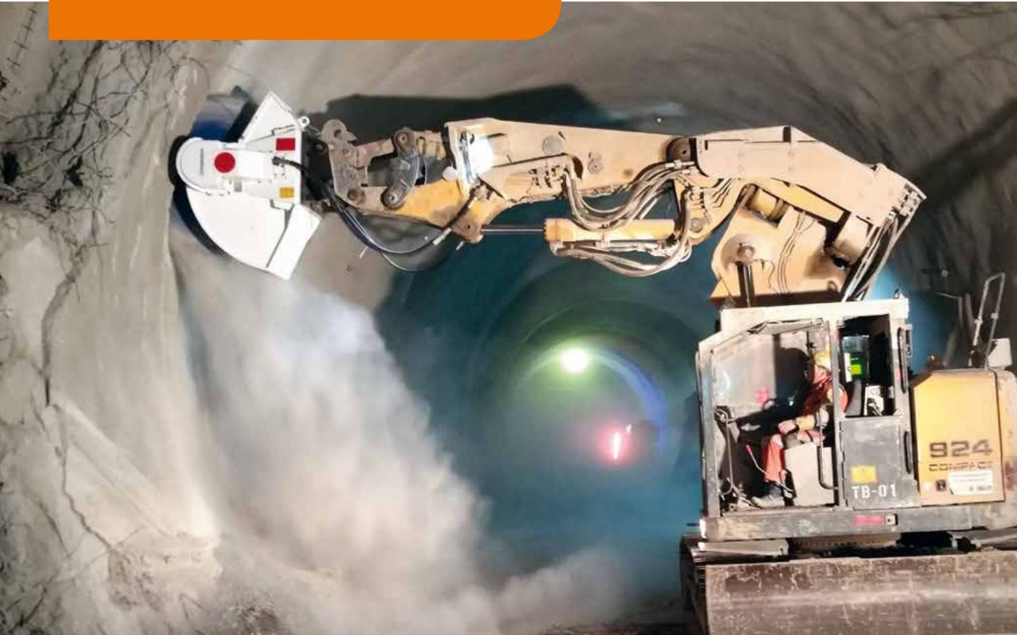
▲ An **EX45HD** planer with tiltrotator removing a 12 cm deep layer from the brick lining in a tunnel. A plastic damp proof layer will be applied to the accurately profiled surface afterwards.
