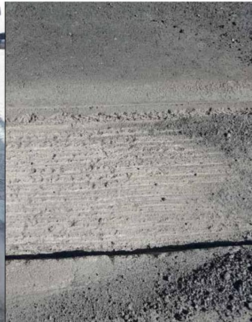
▼ An **EX45HD** with rotation module grinds the hard shoulder of a road. The patch planer milled a strip 45 cm wide by 15 cm deep at a rate of 10 m per minute.
