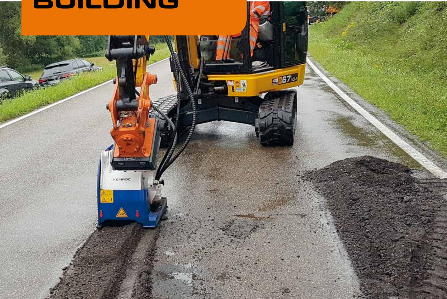
▲ Mounted on a Takeuchi TB 235, this **EX20HD** is removing a 3 cm deep layer of asphalt. The production rate is 25 m<sup>2</sup>/h. KEMROC patch planers produce clean, smooth cut edges.
